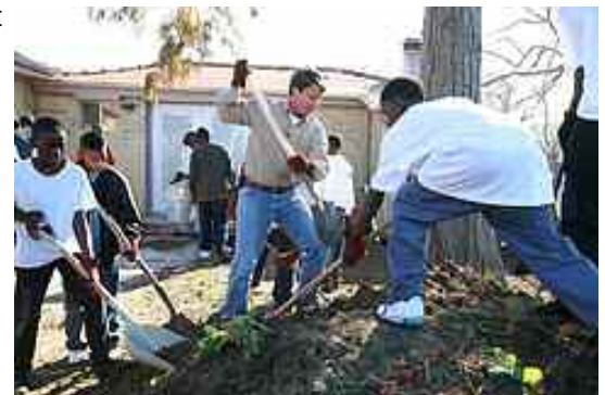
John Edwards volunteers in the yard of a home still being rebuilt from damage caused by Hurricane Katrina.
